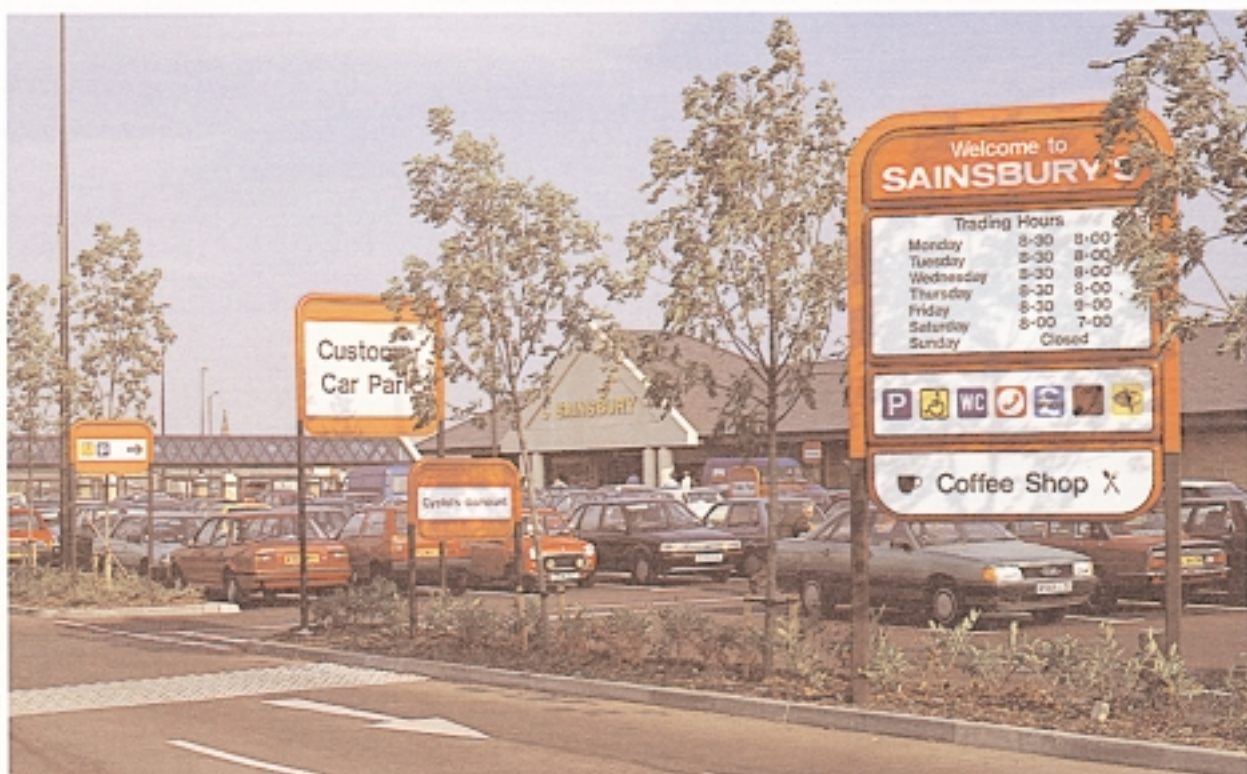
The new Sainsbury's at Leamington, Warwickshire, offers the full range of customer facilities. It replaced a store of less than half its size built in 1971.
