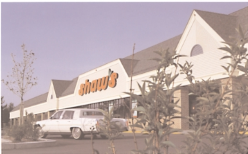
The Shaw's supermarket at Carver, Massachusetts, was one of six new stores opened in New England during the year.
