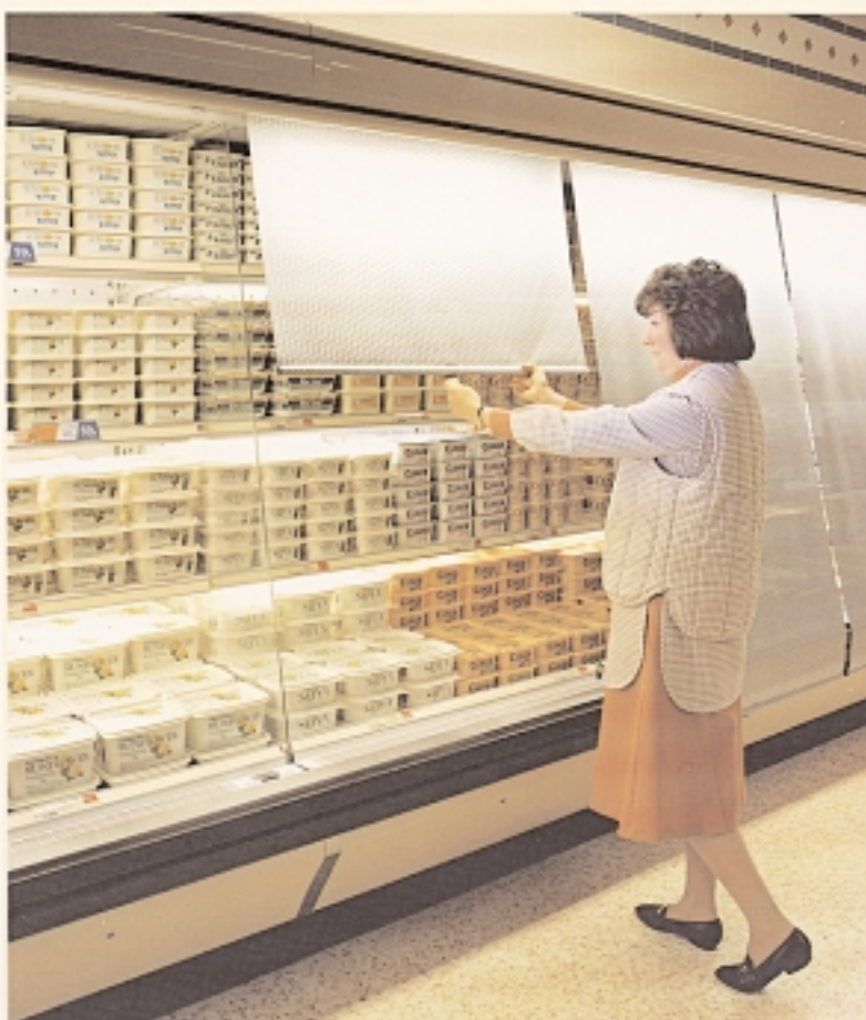
Sophisticated energy-saving systems help save up to £10 million on our annual energy bill and are supplemented by simple techniques such as closing blinds nightly on chiller cabinets.
