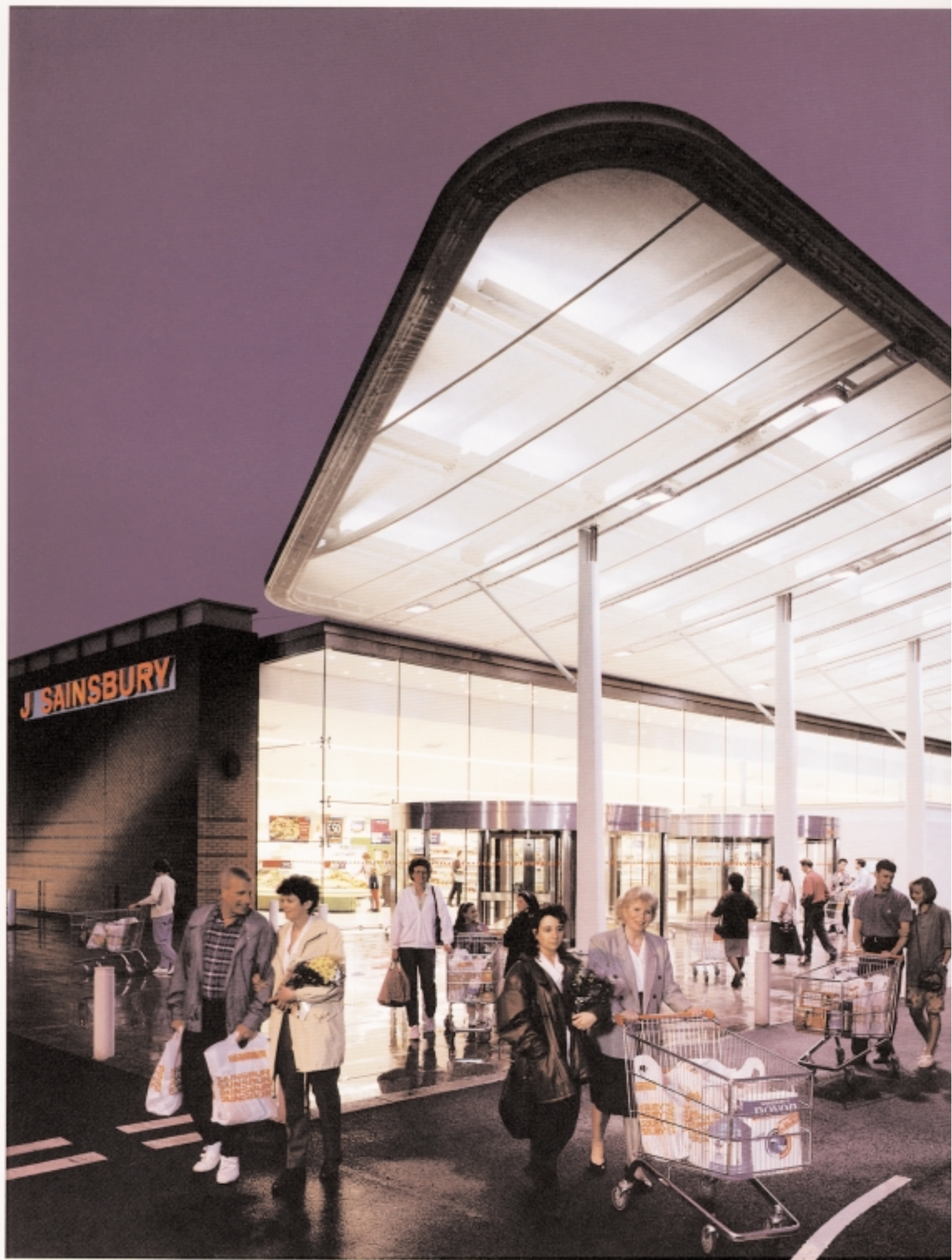
Our store at Canley, Coventry, which opened in November 1993, won the Royal Fine Art Commission and Sunday Times Building of the Year Award 1994 (Commercial Category). Faced in glass, it has a wing-shaped, transparent canopy stretching along the length of the building.
