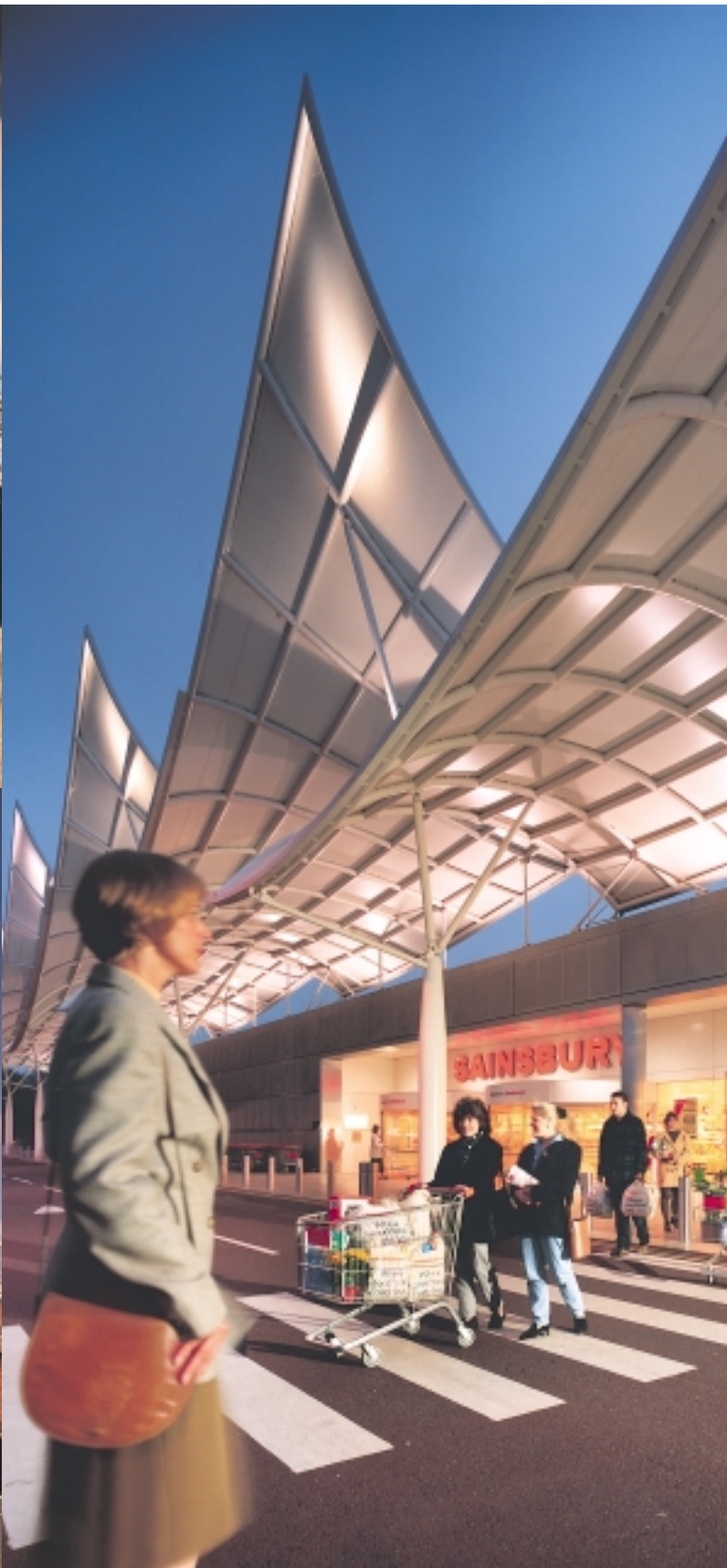
The architecture of our new Marsh Mills supermarket at Plymouth makes it one of the most outstanding stores to be opened last year. The link with the site's maritime associations provides a striking silhouette.
