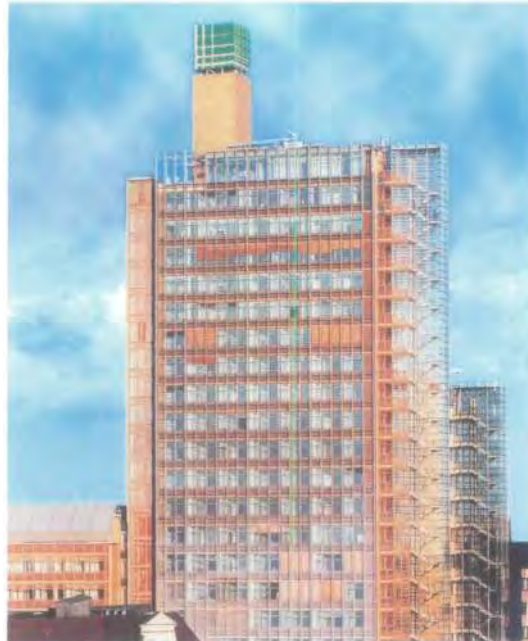
The effect is more than visual: The debis Haus at the Potsdamer Platz is redefining Berlin as a center of communication.
