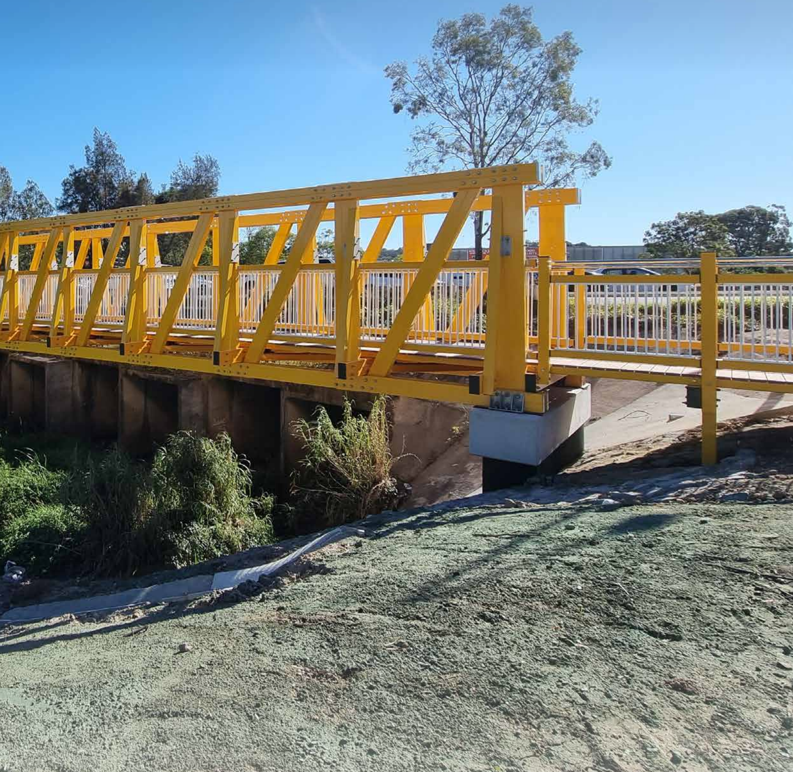
Compton Road Bridge, Slacks Creek, Queensland
