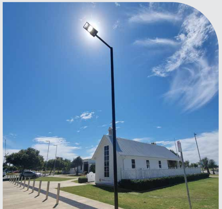
Wagners' CFT manufactured light poles, Southport, Queensland
