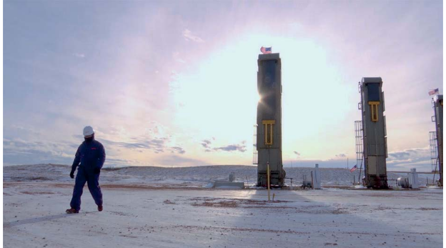
An oil facility powered by Aggreko in North America
