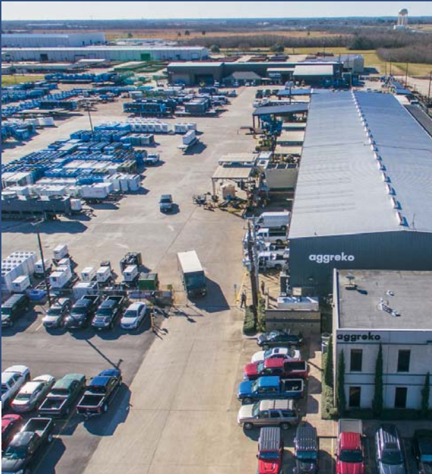
Aggreko's Pearlland facility in Texas, North America
