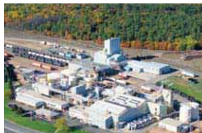
Port Edwards, Wisconsin Facility
