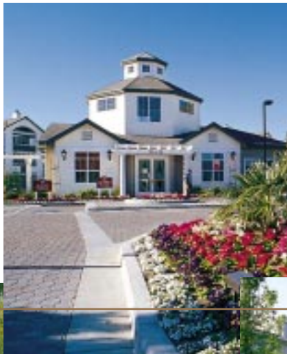
ROSEWALK AT WATERFORD PARK San Jose, CA
