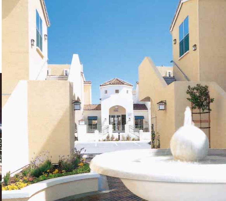
Avalon on the Alameda, San Jose, CA
