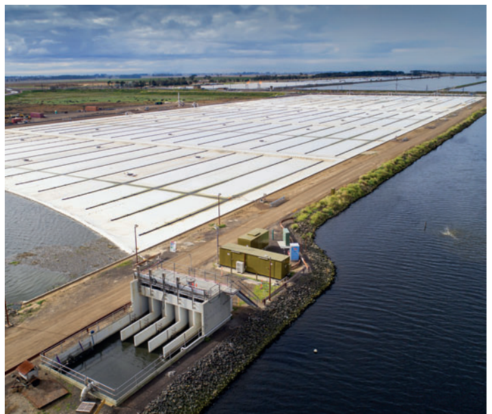
Biogas Collection Cover
