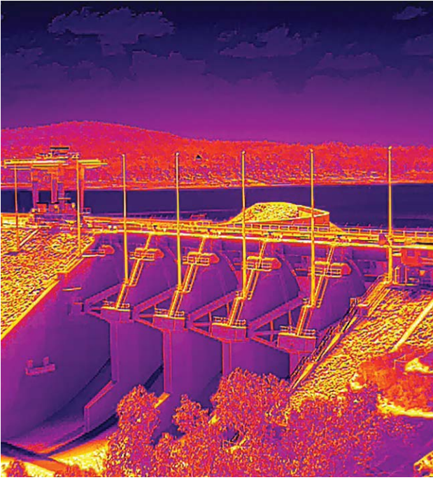
A Thermographic image from the newly deployed inspection UAV where we can analyse temperature differentials in assets.
