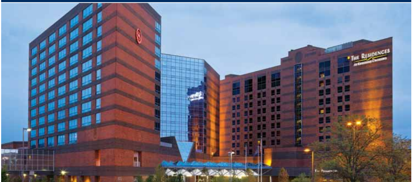
SHERATON INDIANAPOLIS HOTEL AT KEYSTONE CROSSING
