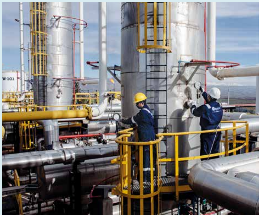
Right: Central processing facility, Taq Taq
