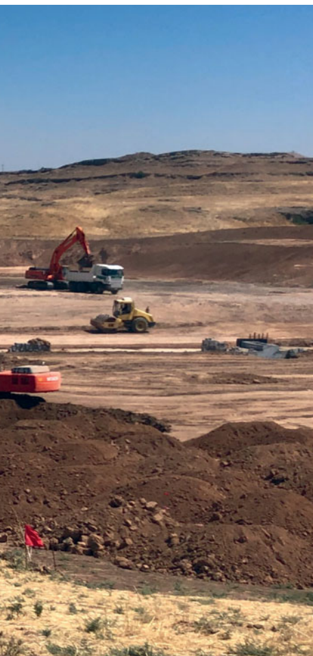
← Work getting underway at Sarta
