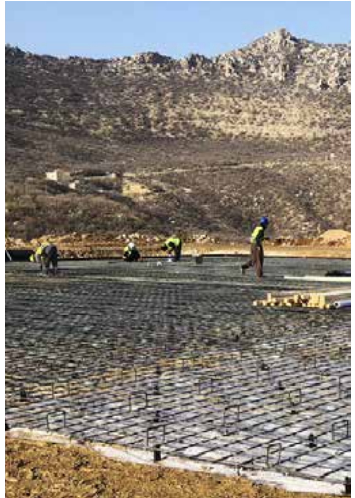
QD-2 well pad construction, Qara Dagh
