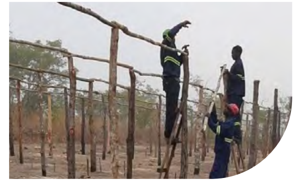
Placing ceiling pillars
