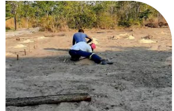
Opening holes for pillars
