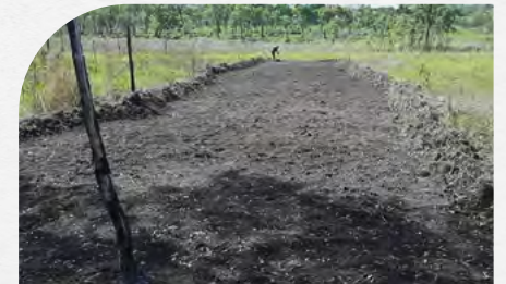
Firebreak opening process
