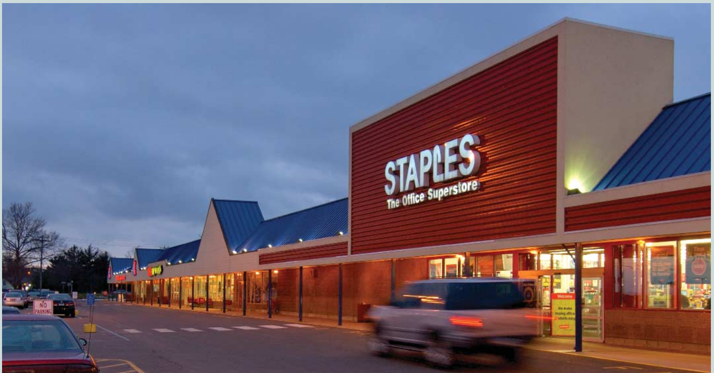
The Dock, Stratford, Connecticut
