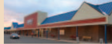
The Dock Stratford, Connecticut
