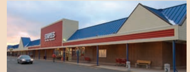
The Dock Stratford, Connecticut
