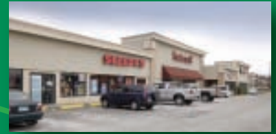
Airport Plaza Danbury, Connecticut
