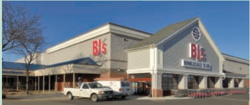
Newly completed BJ's Wholesale Club at The Dock Shopping Center in Stratford, Connecticut
