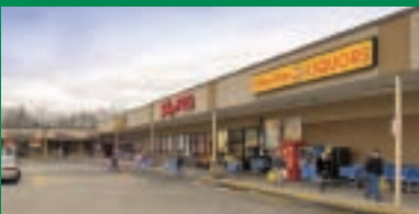
Emerson Shopping Plaza Emerson, New Jersey
