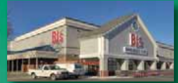
11 The Dock Stratford, Connecticut
