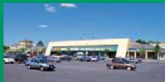
26 Valley Ridge Shopping Center Wayne, New Jersey
