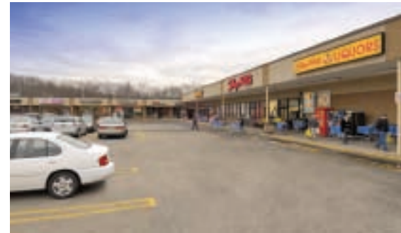
Emerson Plaza 2008 , Emerson, New Jersey
