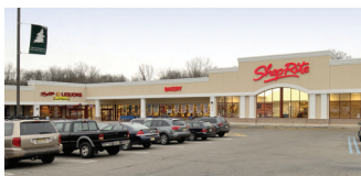
27 Emerson Shopping Plaza Emerson, New Jersey
