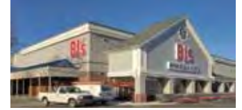
11 The Dock Stratford, Connecticut
