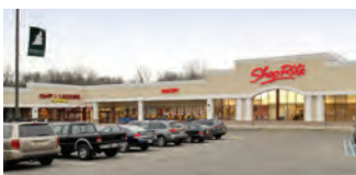
30 Emerson Shopping Plaza Emerson, New Jersey
