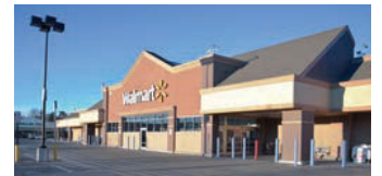
8 New Milford Plaza New Milford
