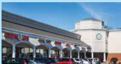
36 Pompton Lakes Town Square Pompton Lakes
