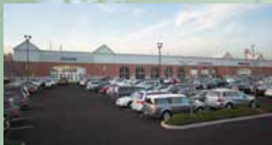
5 Fairfield Centre Fairfield
