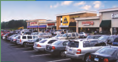
7 Airport Plaza Danbury
