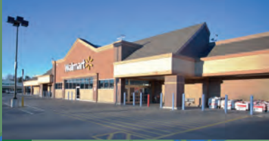
8 New Milford Plaza New Milford
