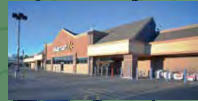
8 New Milford Plaza New Milford
