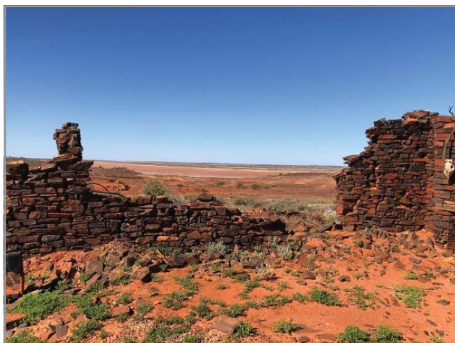
View South through old circa 1900 building, Mainland area, Cue
