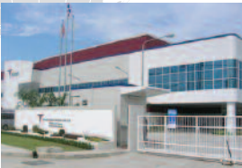
In 2007 Triumph expanded its presence in Asia with the opening of an 85,000 square foot MRO service center just south of Bangkok, Thailand. As the Asia-Pacific headquarters for Triumph's Aftermarket Services Group, the new facility replicates many of the capabilities of Triumph companies in the United States.
