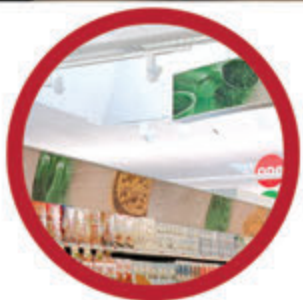
LED Direct & Indirect General Lighting
