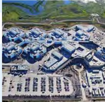
Edmonton Remand Centre Edmonton, Alberta
