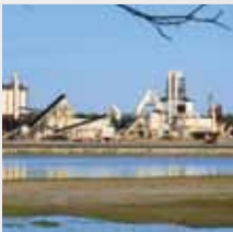
Astec Wood Pelletizing Plant
