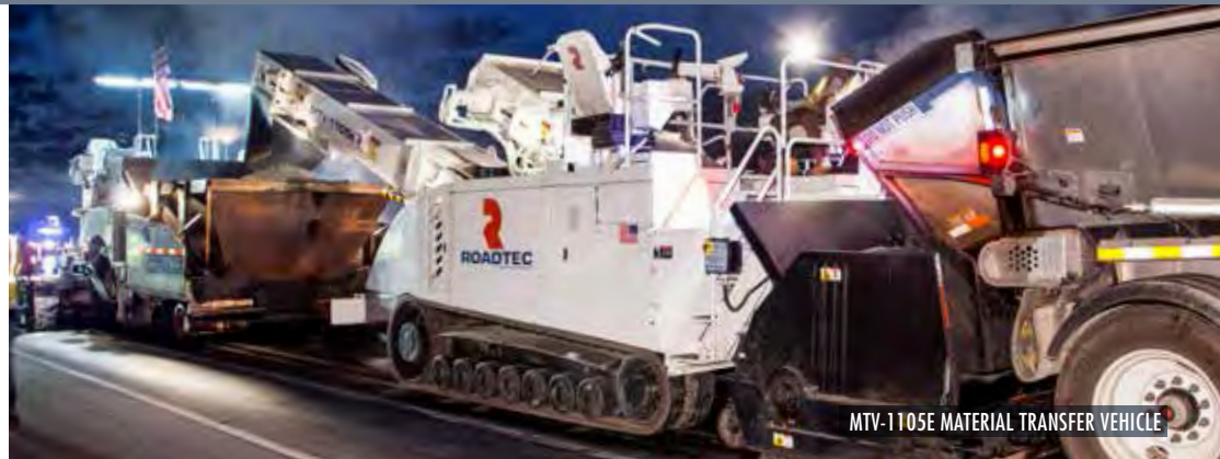
SB-1500E SHUTTLE BUGGY® MTV WORKING WITH RP-195E PAVER
