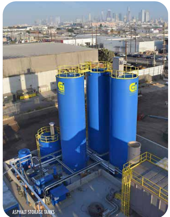
COMBINATION TANK FOR STORING BOTH LIQUID ASPHALT AND FUEL OIL
