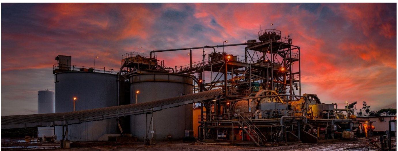
Figure 1: Processing plant post commissioning
