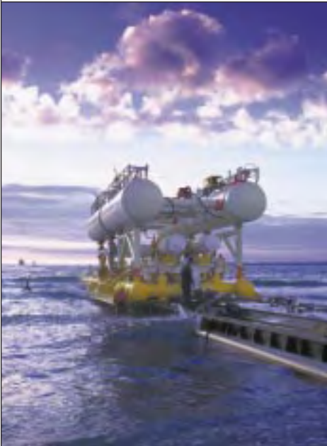
HALLIBURTON SUBSEA places a pre-fabricated offshore pipeline bundle with its Controlled Depth Tow Method.
