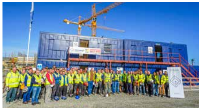
Working Safely Near Utilities - Tool Box Talk at the Glenveagh Rush site.
