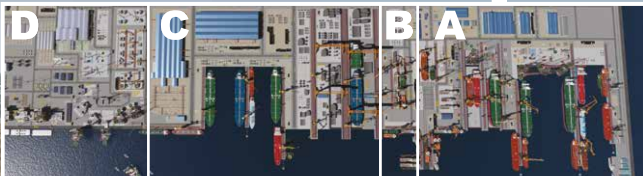
Zone D Technical Partner: Lamprell New build jackups
