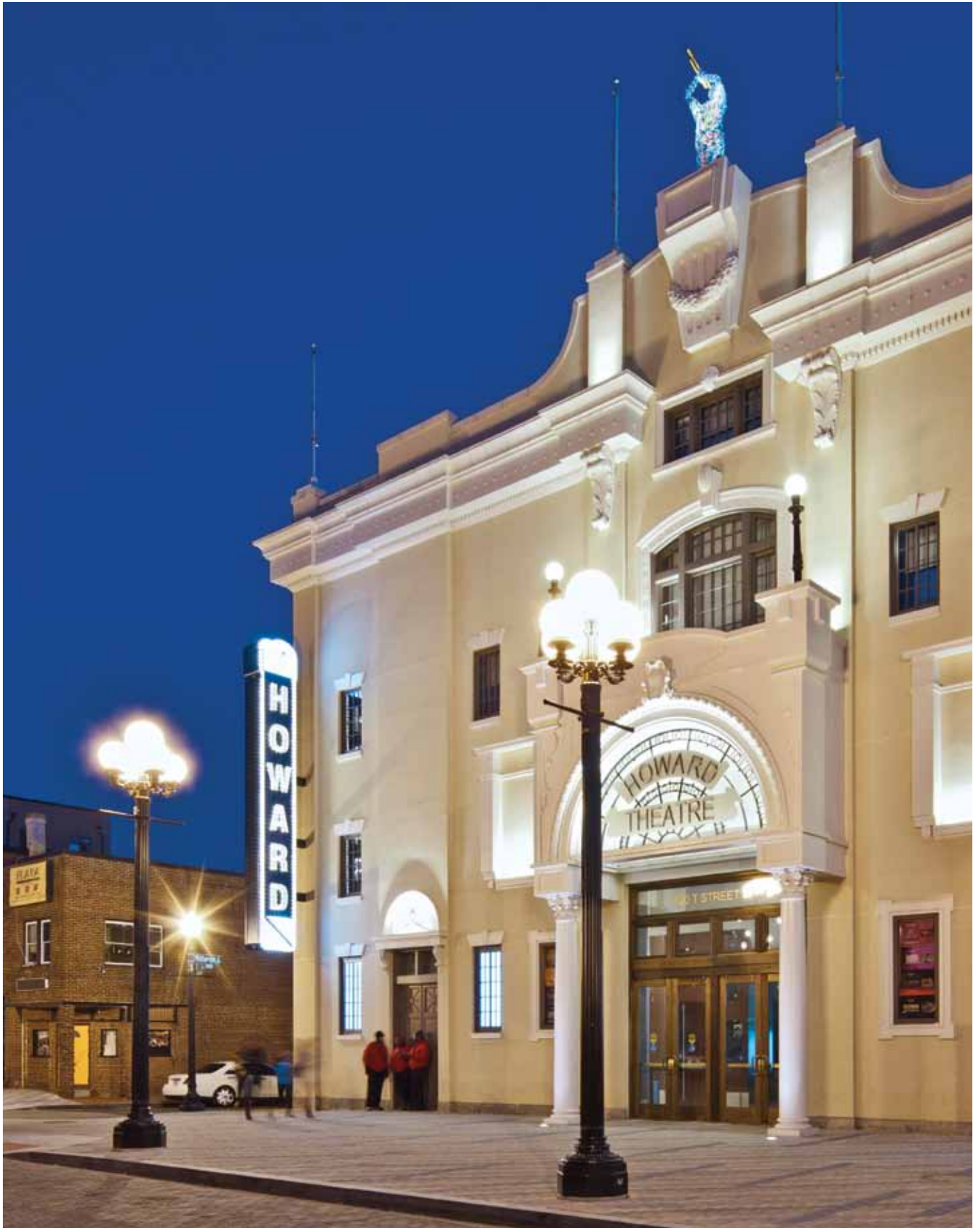
EagleBank client Howard Theatre, Washington, DC. EagleBank helped provide the funding for the restoration of this historic theater in the District's Shaw neighborhood. From Downtown to Georgetown, from Nationals Park to the Potomac River, EagleBank is honored to be a part of Washington, DC's revitalization.
