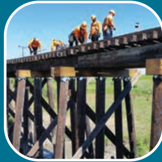
Maintenance and Repair of Railroad Bridges and Structures - North America
