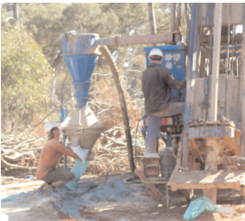
RC Drilling at Wattle Dam
