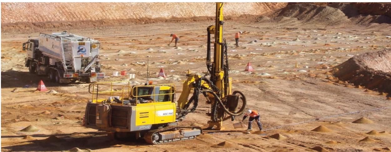
Wattle Dam Drill and Blast
