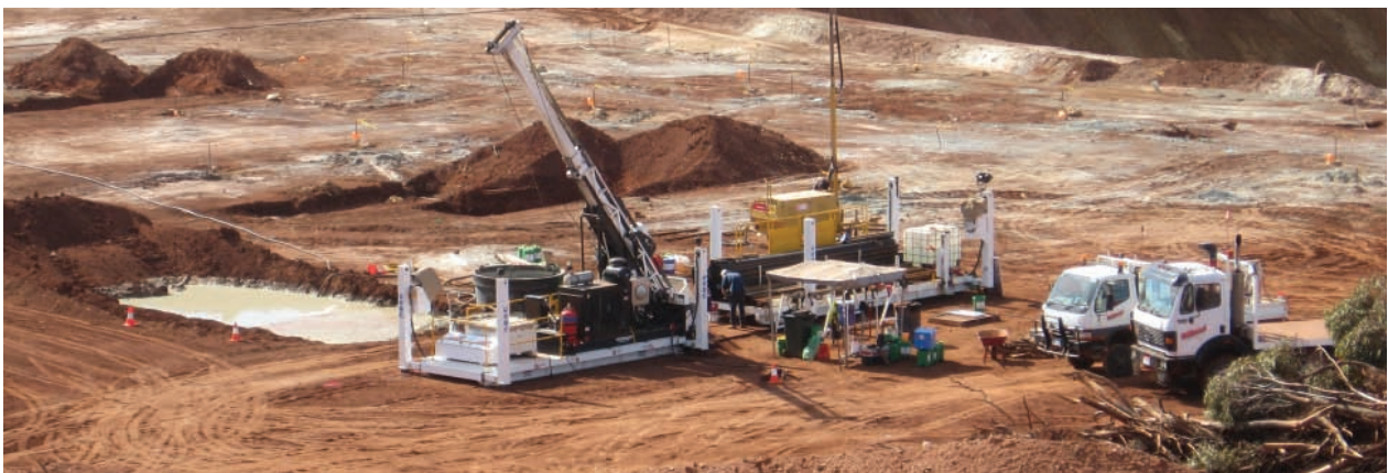
Diamond Drilling beneath Wattle Dam
