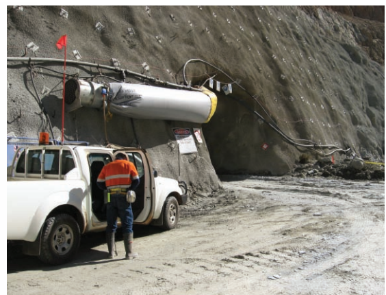
Figure 4A Preparing to go underground
