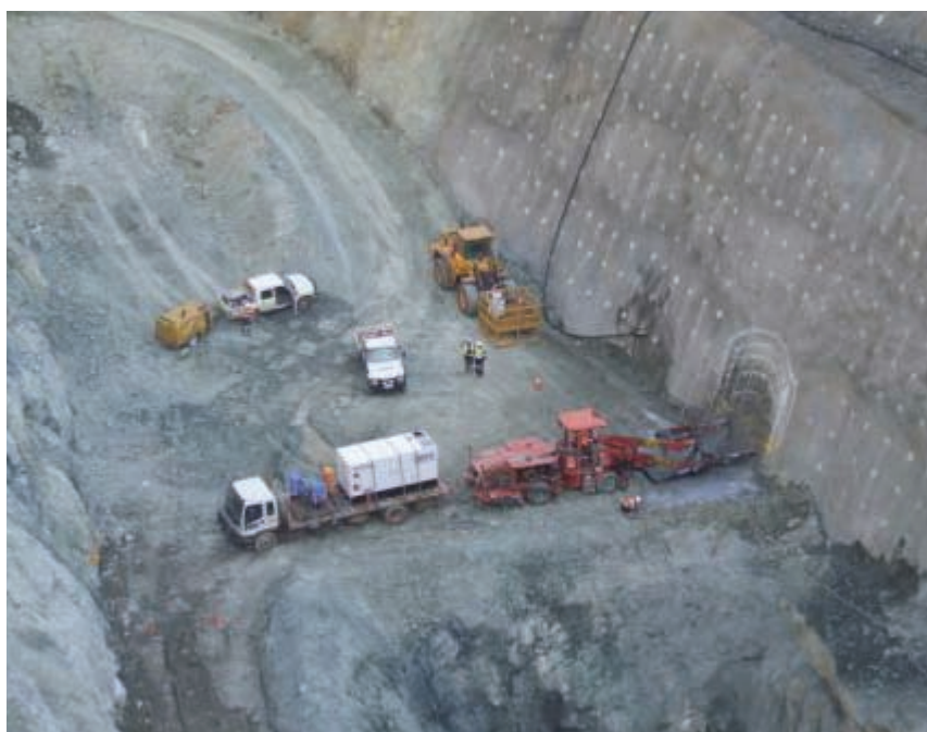
Figure 8 Preparation work for portal development
