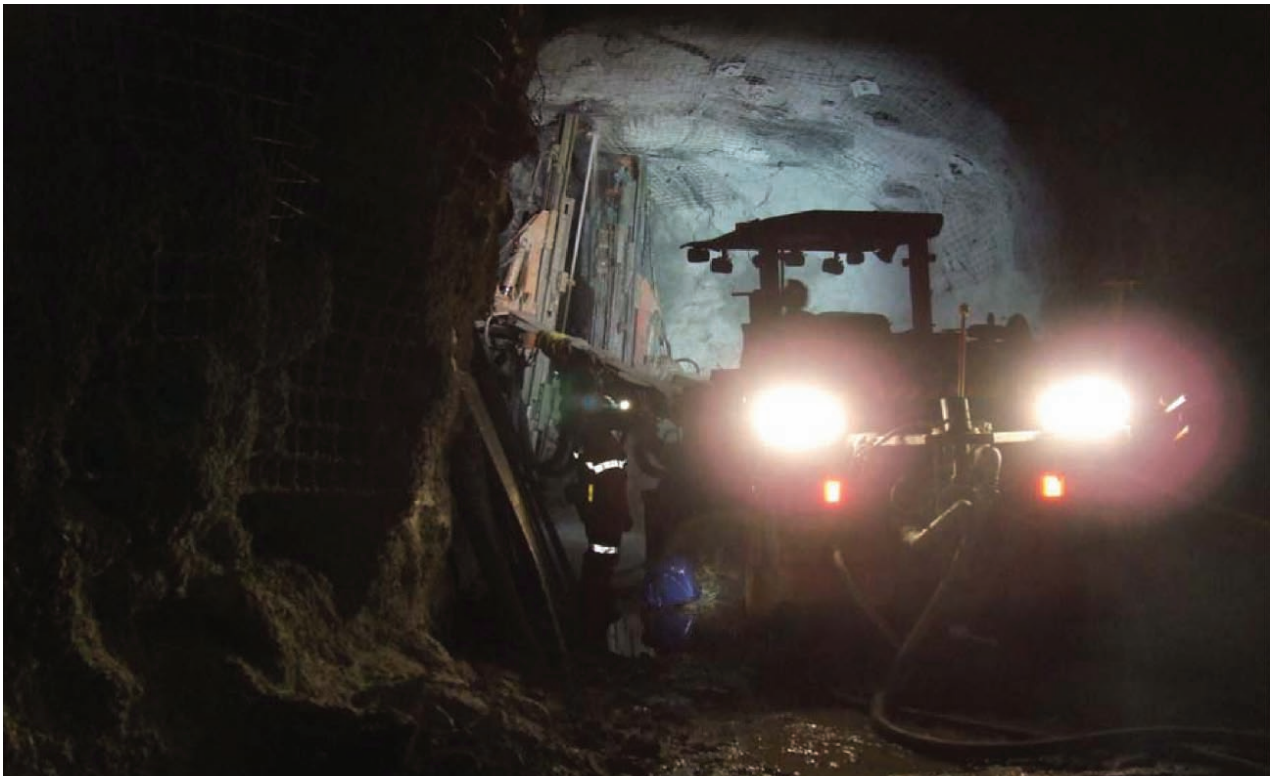
Figure 1 Twin Boom Jumbo underground at Wattle Dam
