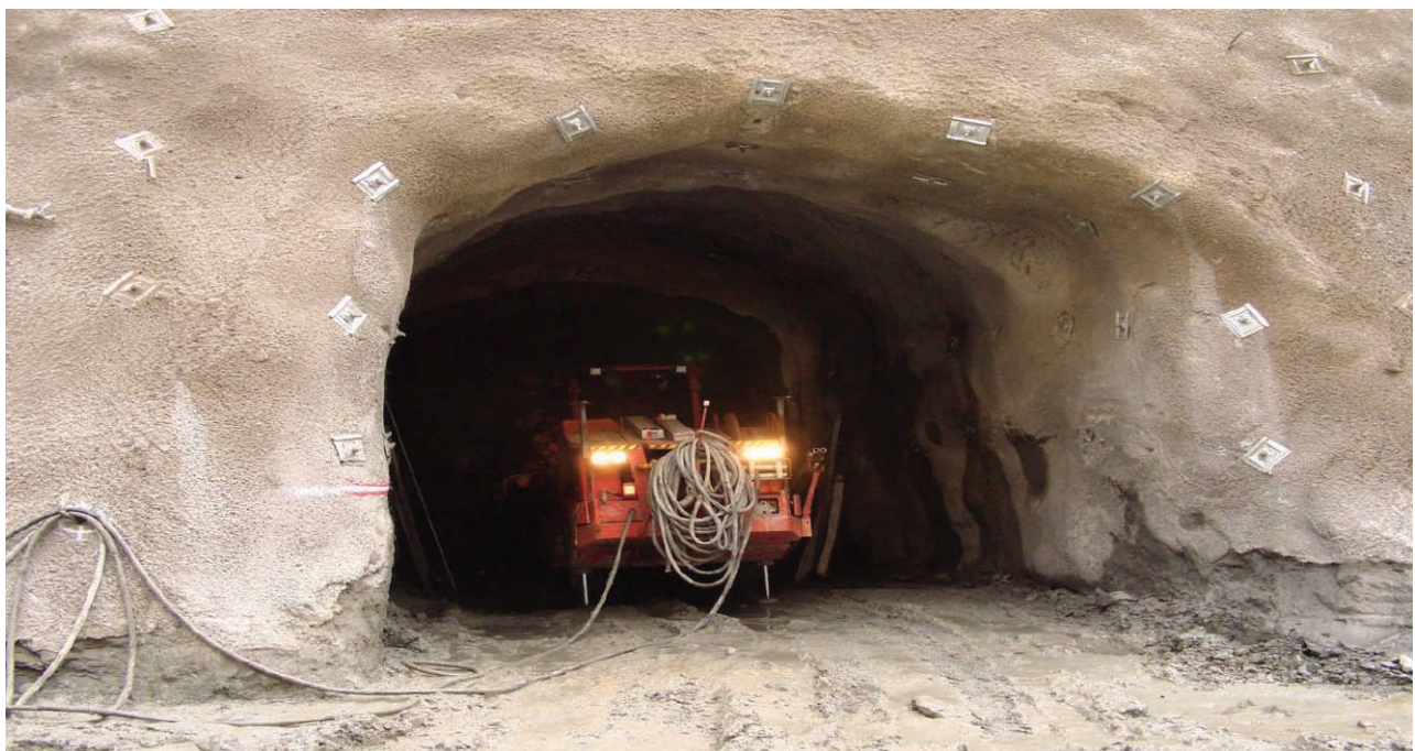
Figure 6 Wattle Dam Mine Portal
