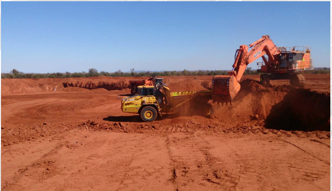
Figure 5: Coogee pit commencement August 2013
