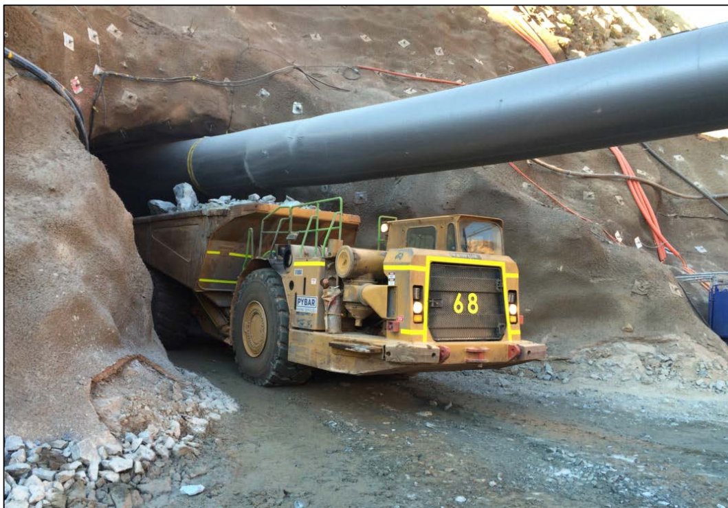
Figure 4: Vivien decline portal
