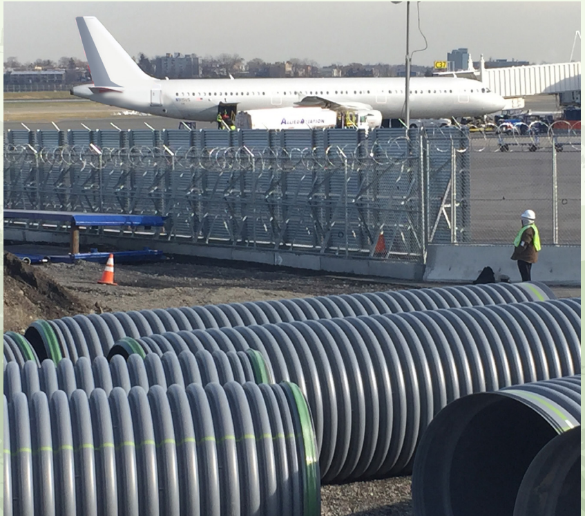
Large diameter HP pipe installation at LaGuardia Airport
